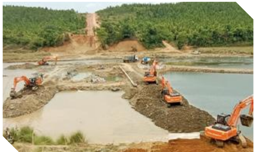
↑ Open Cut Method- Dhobi Durgapur pipeline project
