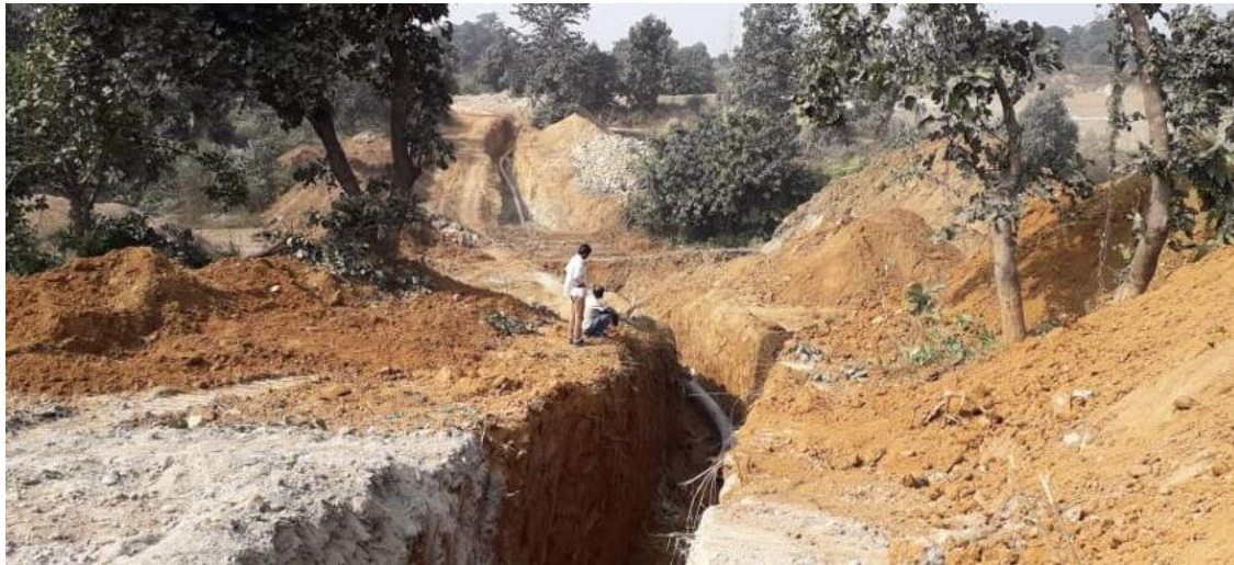
Pipeline laid for a Cross-Country Project
